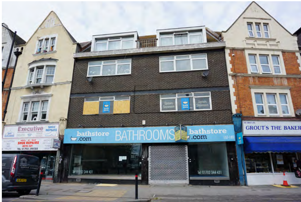
Poor quality rebuild on the site of an historic building at Nos.179-181 Hamlet Court Road
