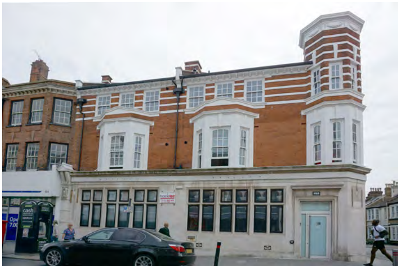
Former bank at No.152-154 with original shop front
