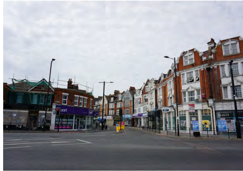
02: Focal point of Nos.205-211 Hamlet Court Road, with views round the sweeping curve of buildings
