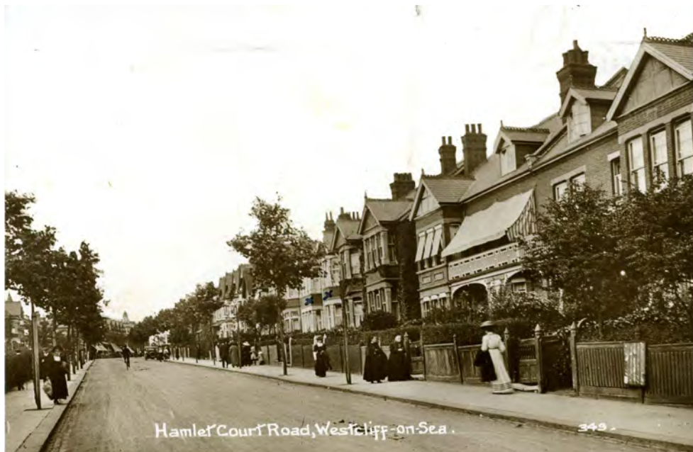
The east side of Hamlet Court Road looking north, with properties that were originally residential with front gardens. Reproduced with the kind permission of the Hamlet Court Conservation Forum
