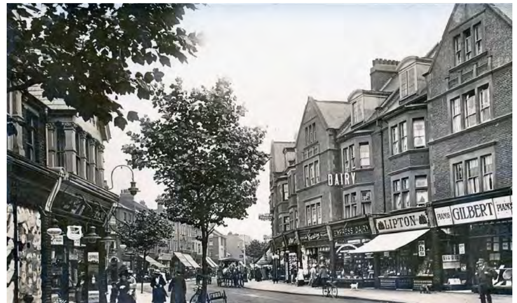
Historic photograph showing the Conservation Area with trees lining one side of the street
