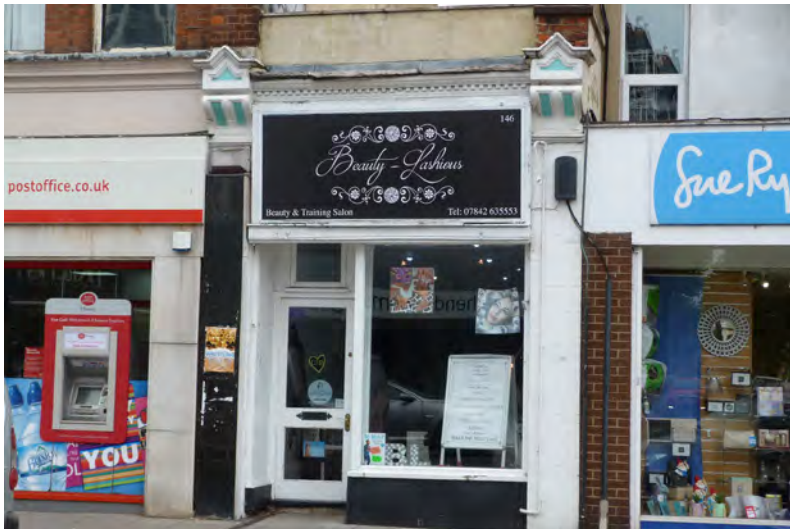
No.146, Now Charisma Hair Xtensions', with a largely intact original shop front
